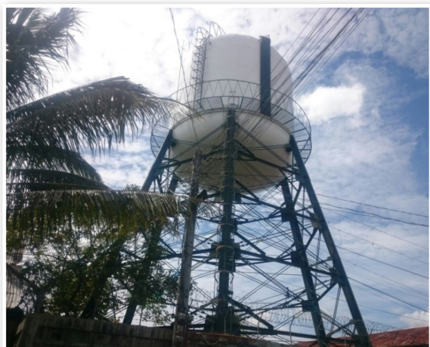
Resettlement Elevated Reservoir
